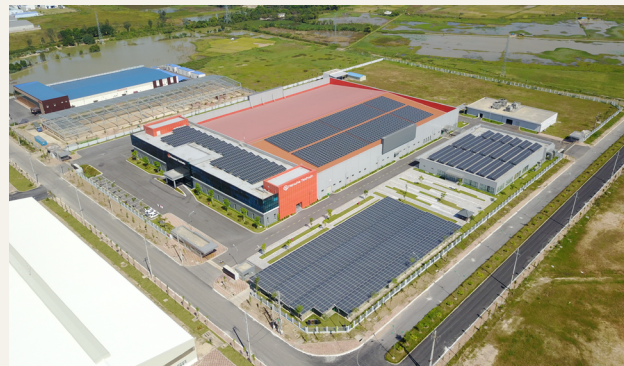
Solar Panels at Hanwha Vision Vietnam
